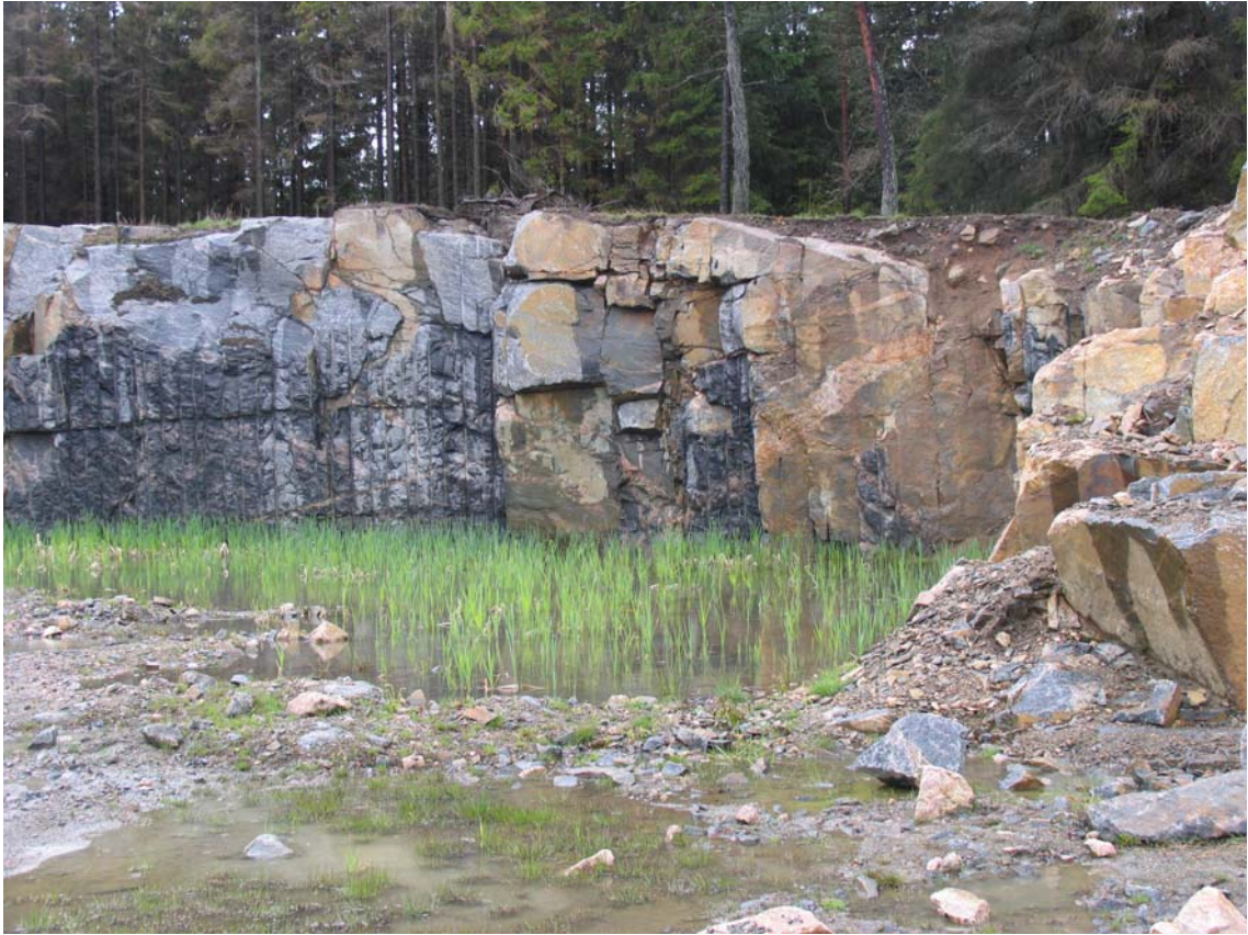
Figure 18. Section from Præstebo quarry with vertical and horizontal fractures. The spacing of the vertical fractures is changing from very small (cm size) to a spacing of several metres. Only one horizontal fracture is seen in the approx. 3 m high section.
