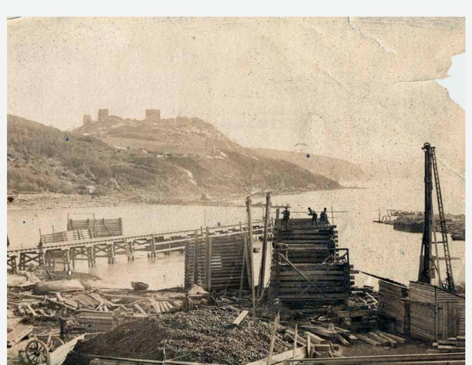
Hammerhavn harbour was constructed in 1890-1892. The photo shows cofferdams in the process of being built.
